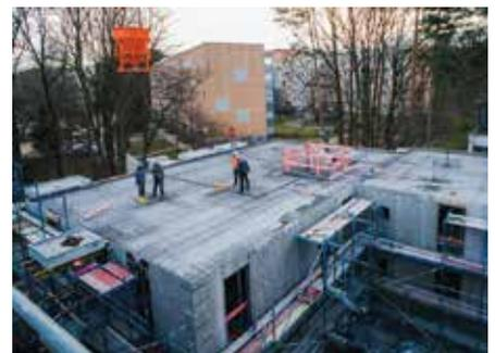
**Fig. 5:** VST panels are used for floor formwork as well as wall formwork. The panels are supported using the same propping systems as used with conventional formwork panels
