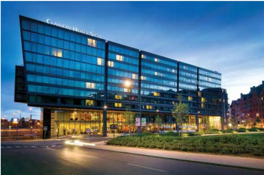
**Fig. 1:** Clarion Hotel Sign, Stockholm, Sweden, built in 2005 using 18,335 m<sup>2</sup> (197,360 ft<sup>2</sup>) of VST wall formwork and 19,165 m<sup>2</sup> (206,290 ft<sup>2</sup>) of VST slab formwork
