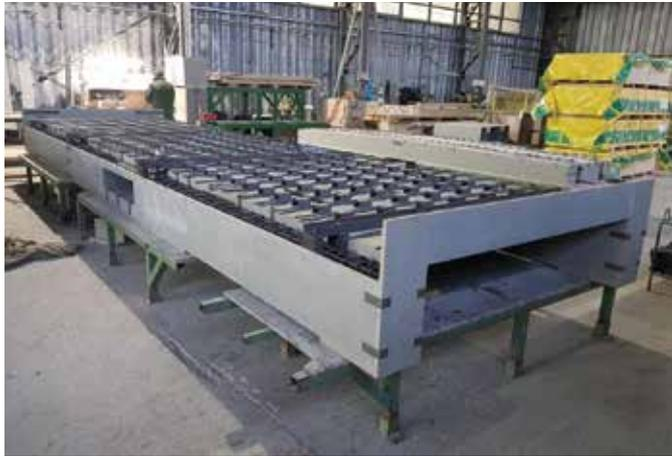
**Fig. 6:** The VST formwork system can be used to optimize processes beyond concrete construction. Here, a prefabricated corridor formwork assembly is being prepared for installation of ventilation ducts, piping, and electrical and communications conduits—all in a controlled environment. In the field, the systems will be connected to adjacent assemblies, minimizing overhead work
